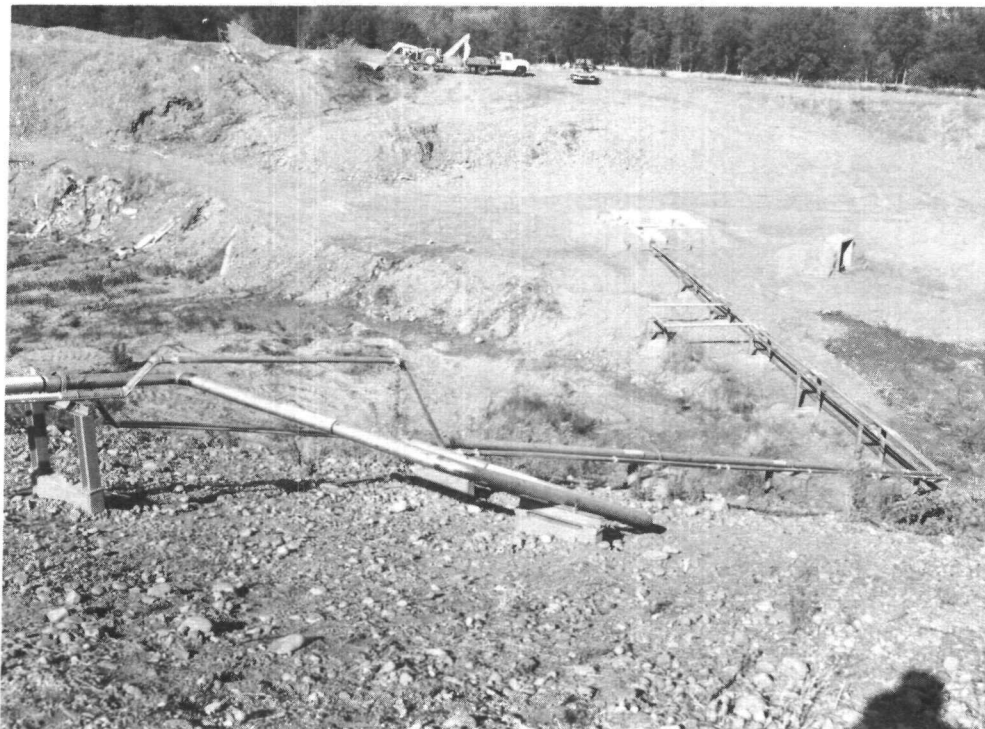
Figure 2 Scale Model Burn Pond, Piping and Pond
