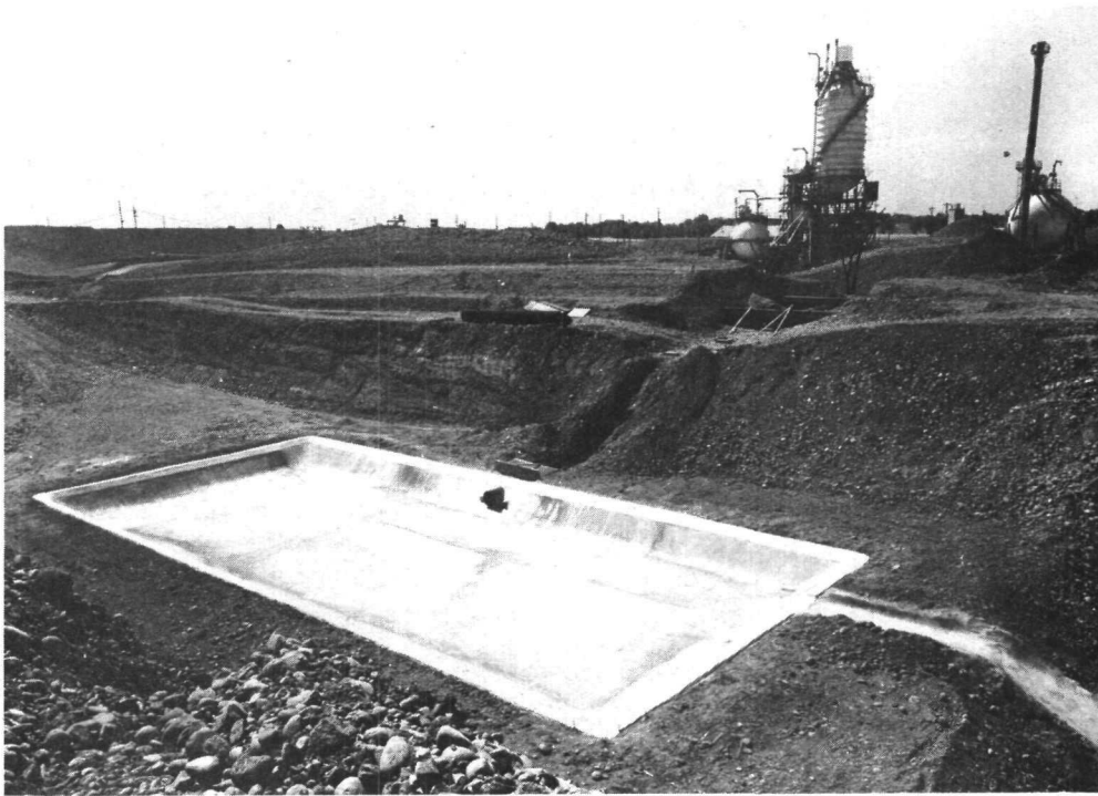
Figure 5 Full-Scale Hydrogen Burn Pond
